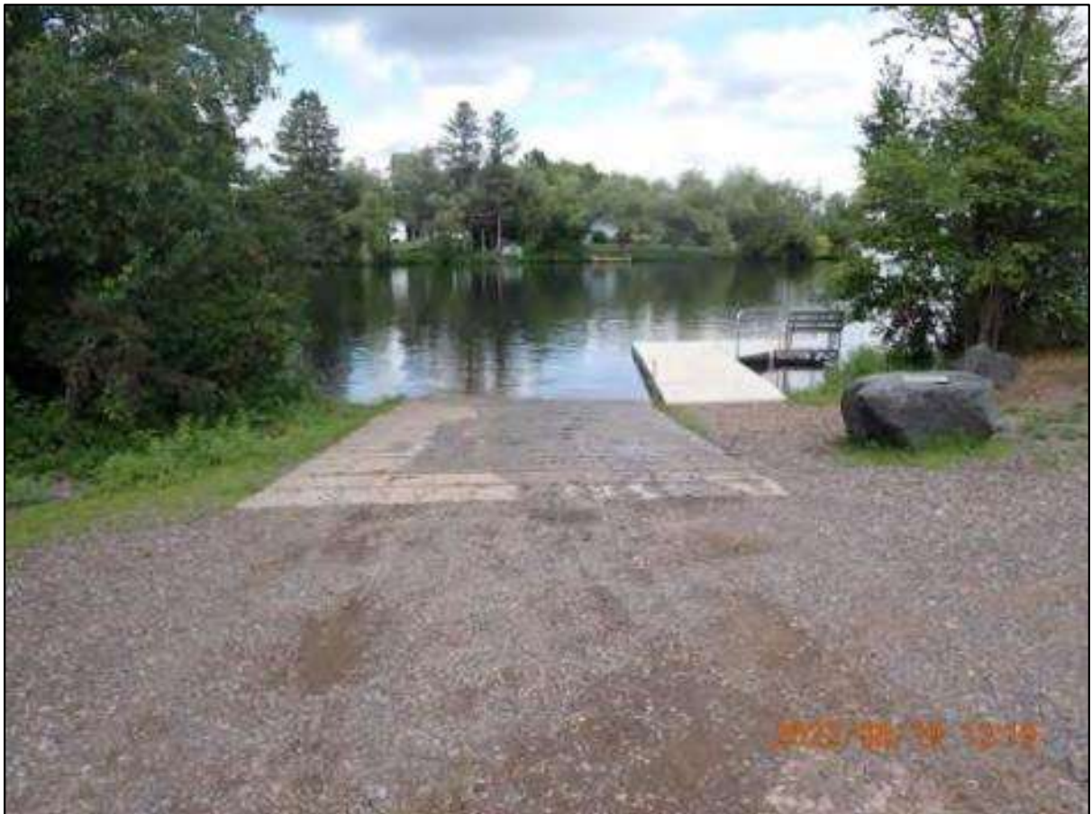
Figure 4.8.1.4.1-4 Hayward City Boat Landing and Dock on Lake Hayward
